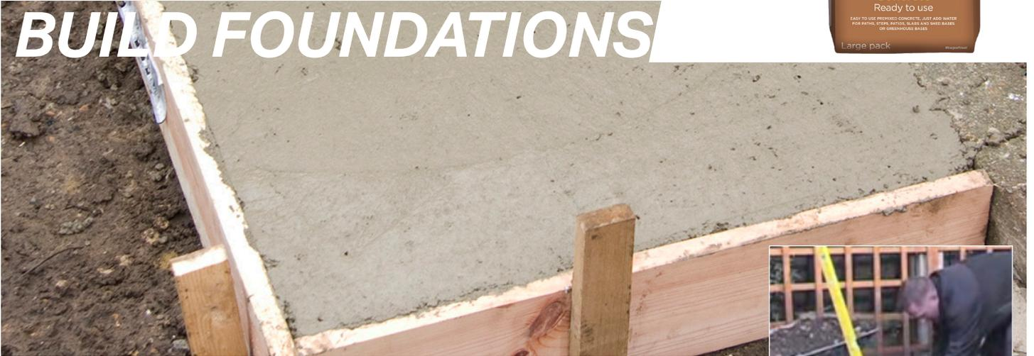
1. Mark the layout of the wall with stakes and dig a trench for the footings down to firm and level ground. The width should be three times the width of the wall.
