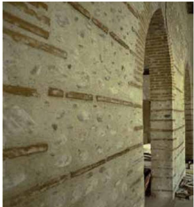
Historic internal wall repaired with Natural Hydraulic Lime mortar
